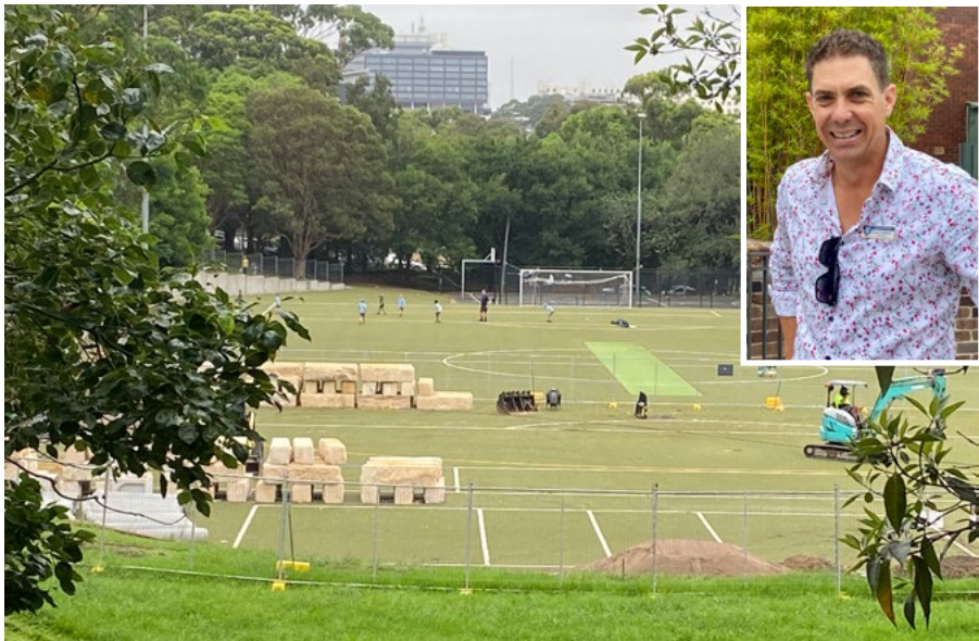
Renovation work at Thomson Park Oval
