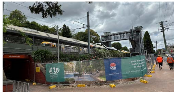
Artarmon footpath and streetscape upgrade currently underway
